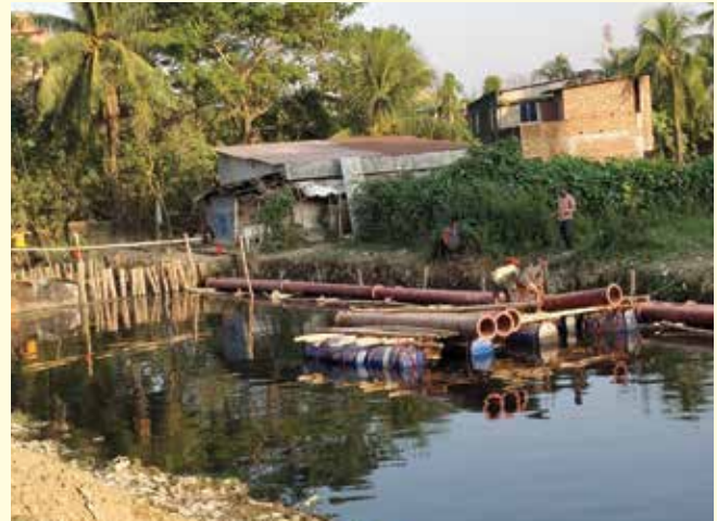
Ongoing Physical work at Noa Khal, adjacent to Noa-Mirza Confluence
