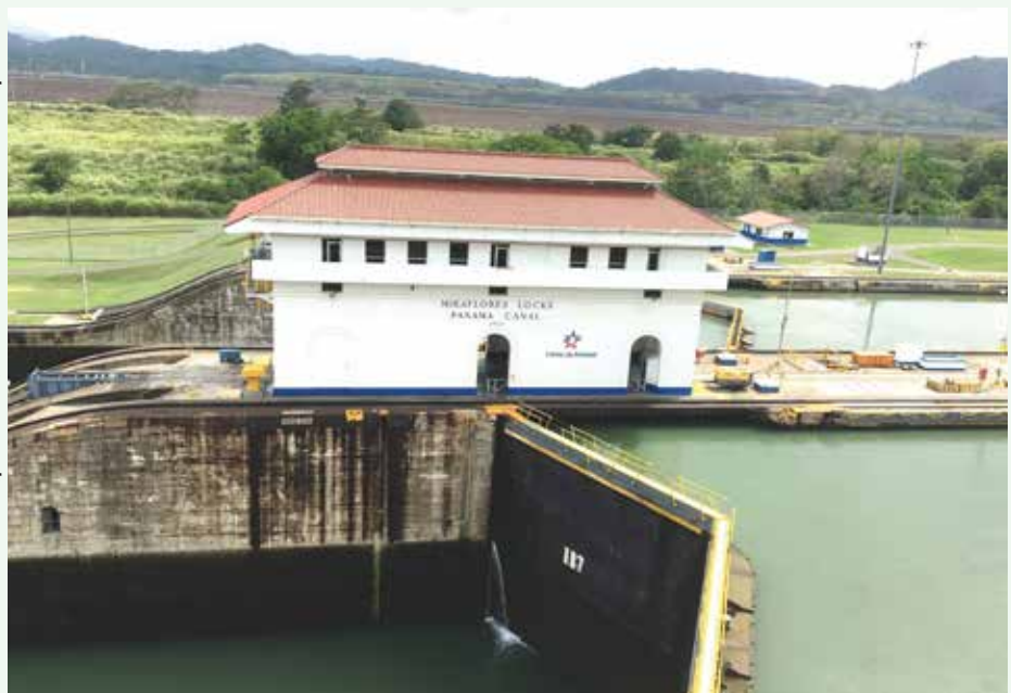
Navigation Lock at Panama Canal, Panama City
