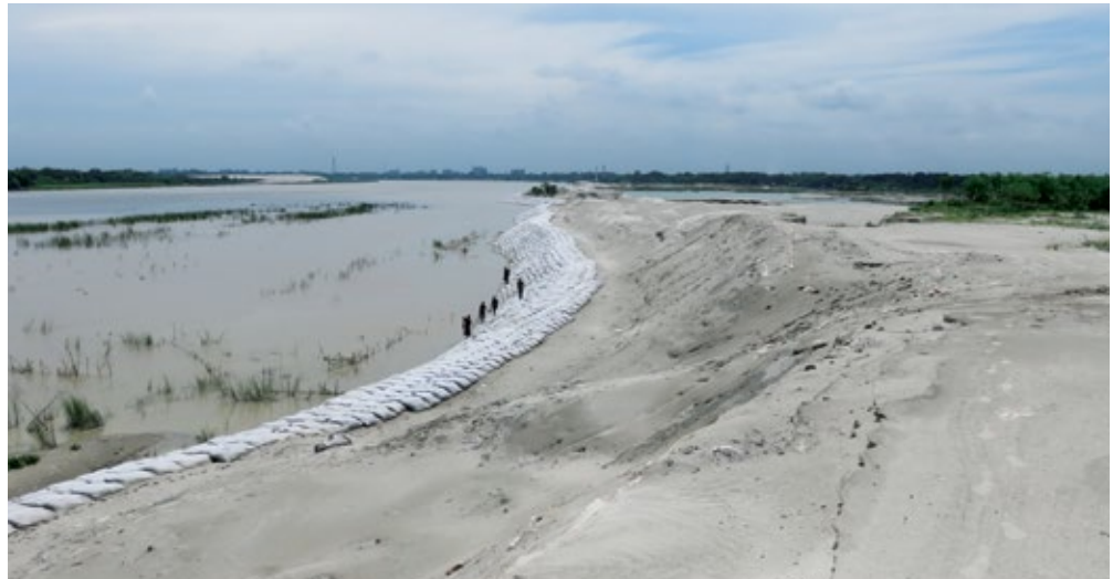
Bank protection along the bank of the Gorai River
